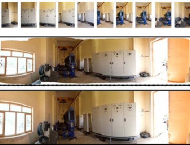
Figure 12. A Sample of multiple sequential images stitching and rectifying
