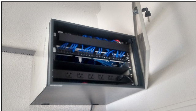
Figure 6. Horizontal Cabling Bracket.
