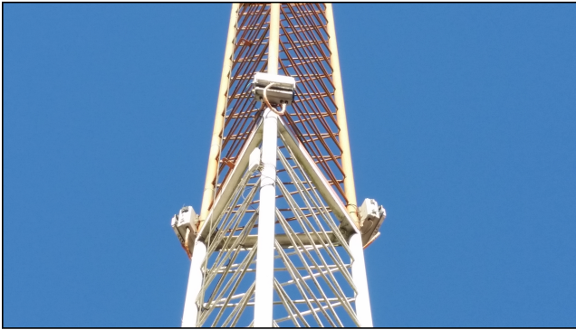
Figure 8. Partial view of the distribution tower with access points.
