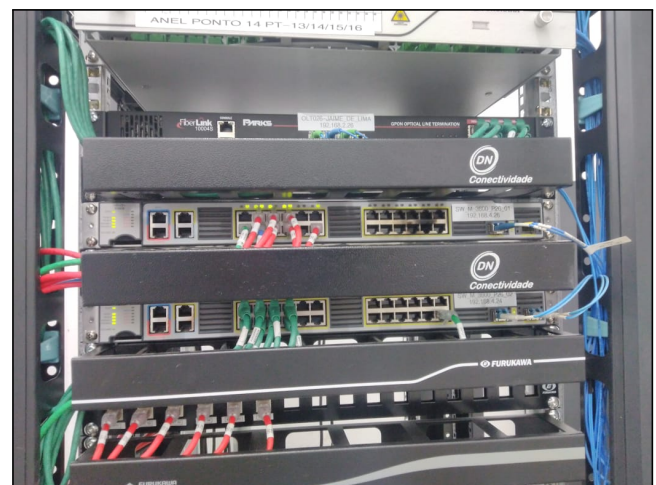
Figure 4. Core switches and OLT installed in the equipment rack.
