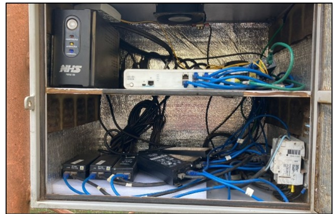
Figure 7. Hermetic box with equipment supporting the distribution tower.
