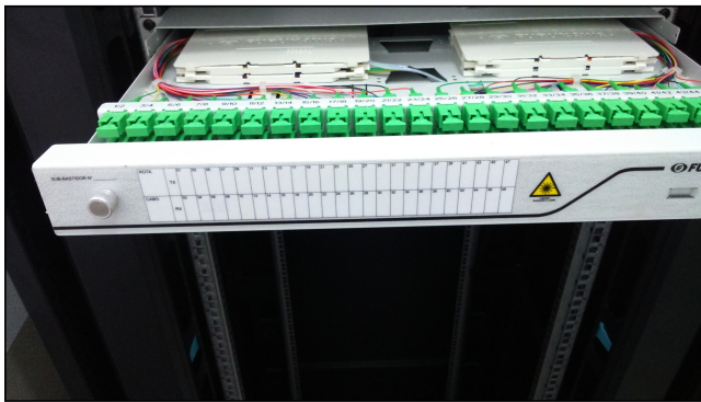
Figure 5. Internal Optical Distribution Frame (DIO).
