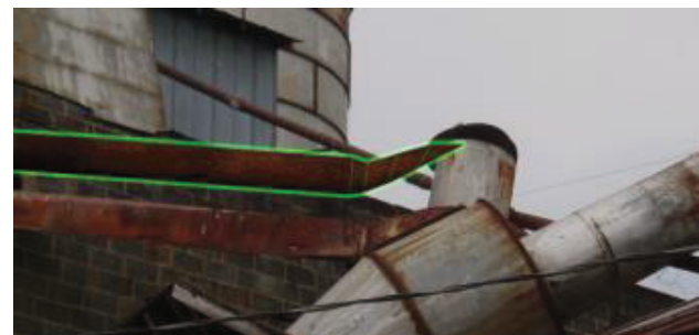
Fig. 25. Corrosion inspection application scenario.
